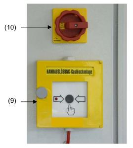
Main switch (10) of the gas detection system and manual release (9) of the fire suppression device (example illustration)
