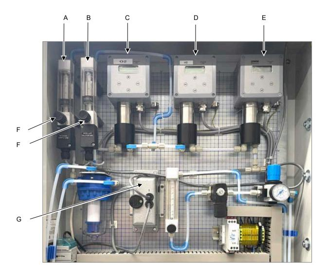
Figure 12: Components of the gas detection
