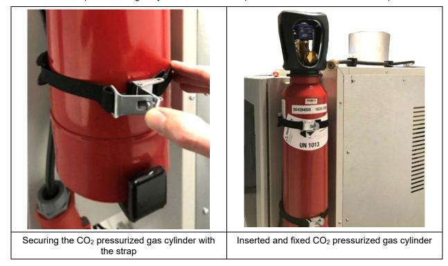
Figure 31: Securing the CO<sub>2</sub> pressurized gas cylinder
