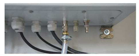
Figure 24: Connection for inert gas at the bottom of the safety module
