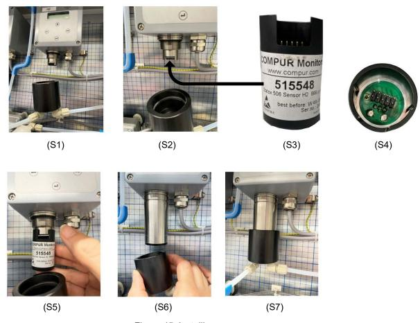
Figure 45: Installing a new gas sensor
