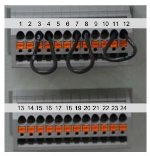
Figure 39: Terminal assignment
