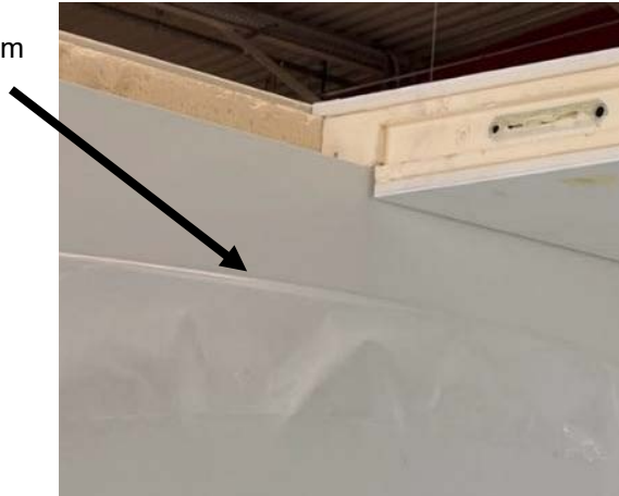
Figure 10: Partially removed protective film during assembly of the wall elements
