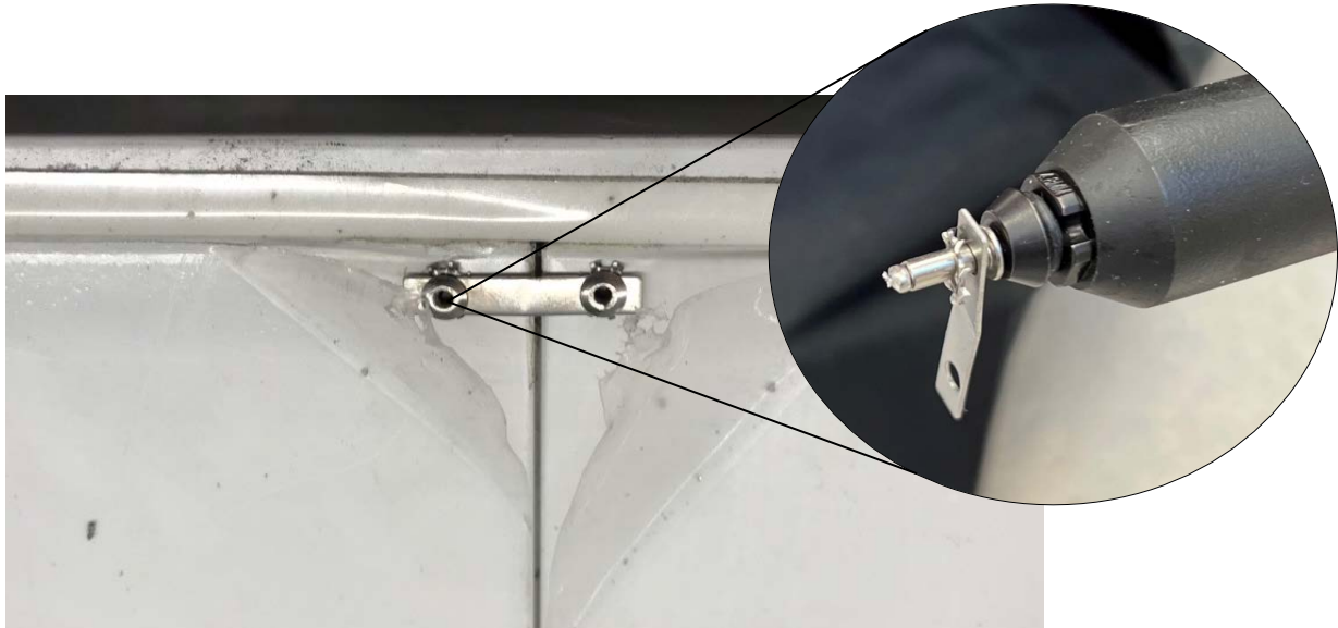
Figure 16: Connection of the ceiling elements
