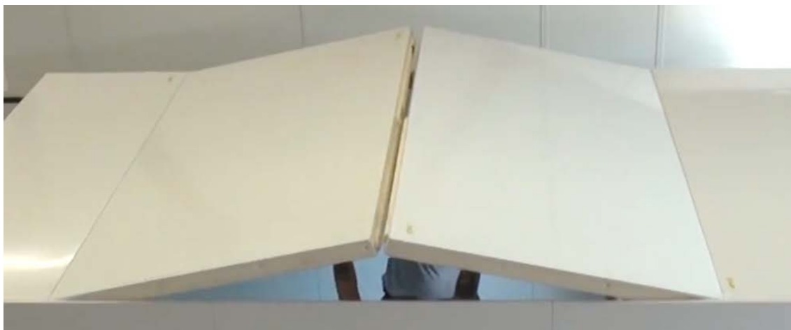
Figure 15: Assembling the last ceiling elements
