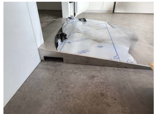
Figure 23: Installing the door sill ramp
