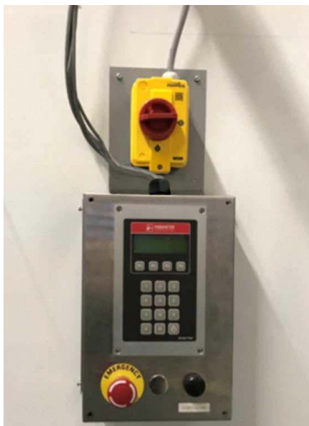
Figure 59: Main power switch mounted above the controller box (View without cover)
