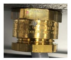
Figure 7: Cable gland with Ex classification
