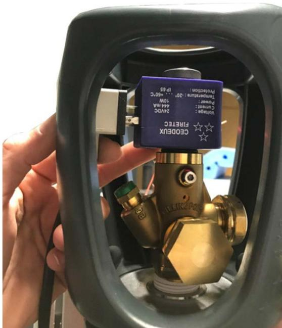
Figure 32: Connecting the coil connector
