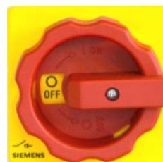
Figure 11: Gas detection system main switch (OFF position)
