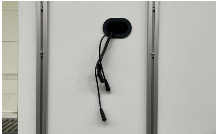
Figure 16: Cables from the distributors of the LED light bar cables, led through the elongated access port to the outside
