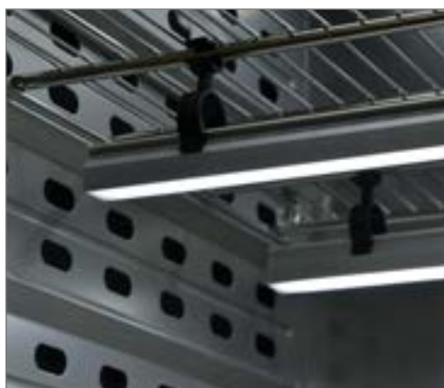
50 cm light bars, fastened to the rack with plastic clips
