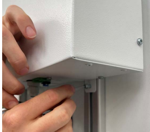
Figure 13: Screwing the CO 2 control box
